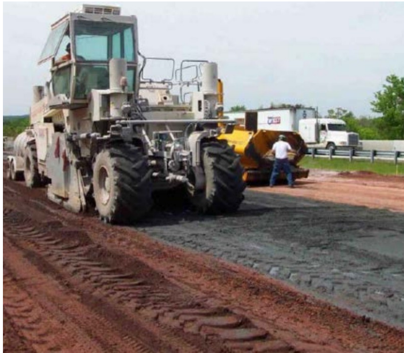
Figure 1: Soil stabilization using FA
